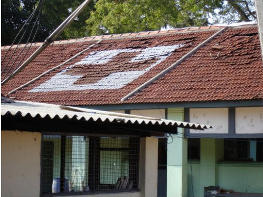
Photo A-1: PTK Hospital Damaged Roof
