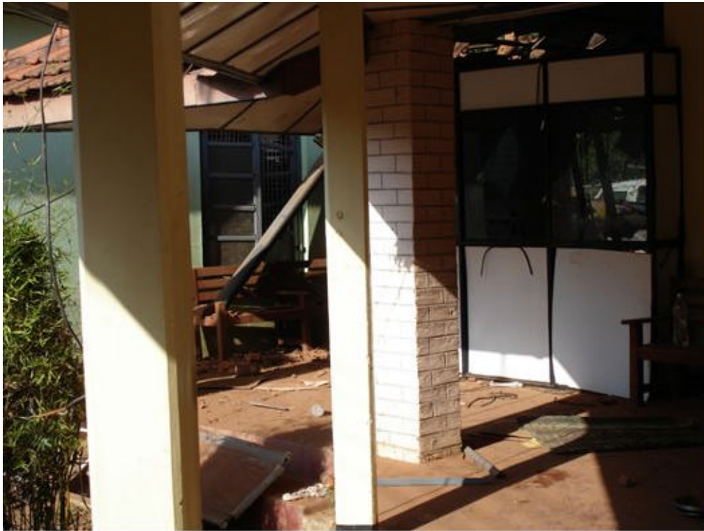
Photo A-3: PTK Hospital Passage Ways
