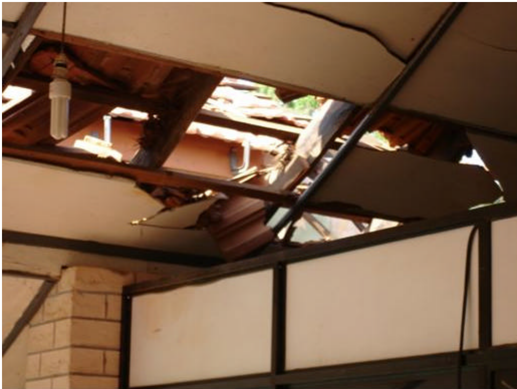
Photo A-4: PTK Hospital Ceiling
